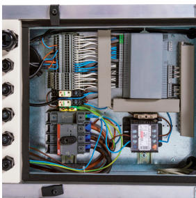
Integrated control Integrated electronic control, inside the unit.
